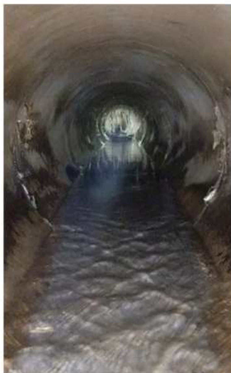
CCTV draining pipe assessment prior jet blasting
