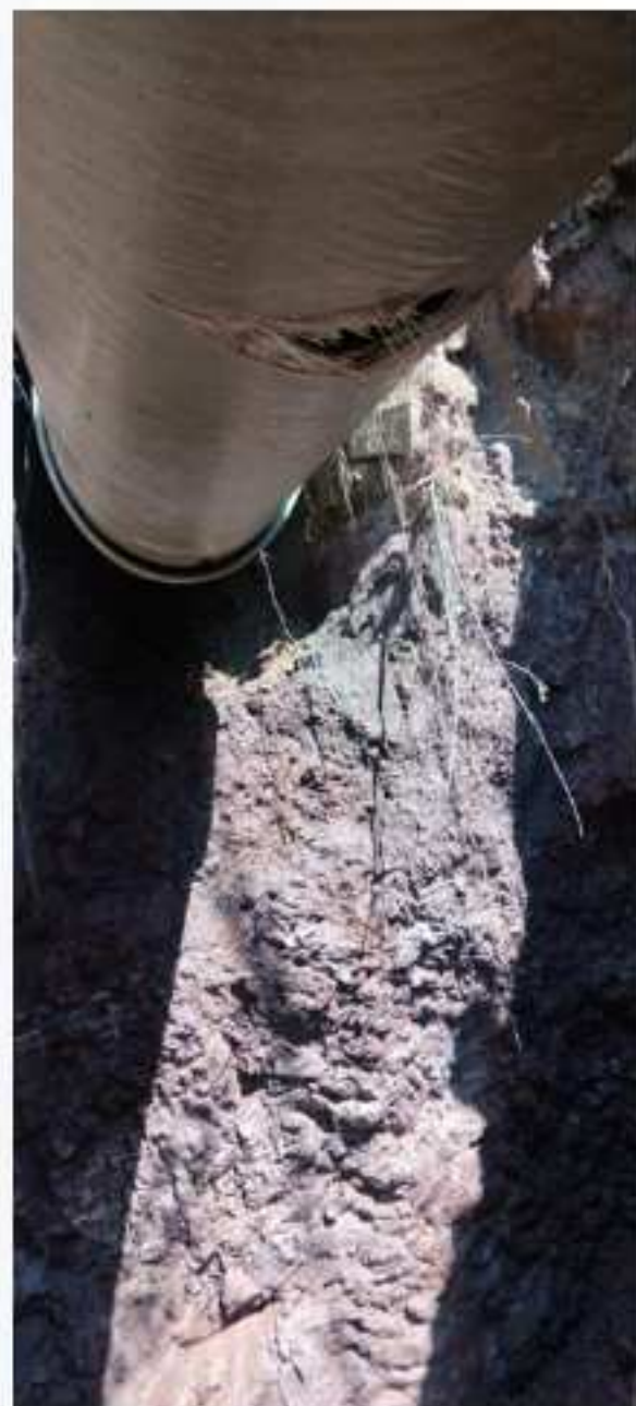
Repairing the GRP main supply line leakage
