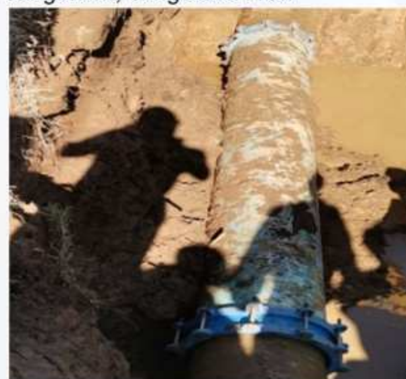
Leaking 400 mm AC pipe replaced with a UPVC pipe
