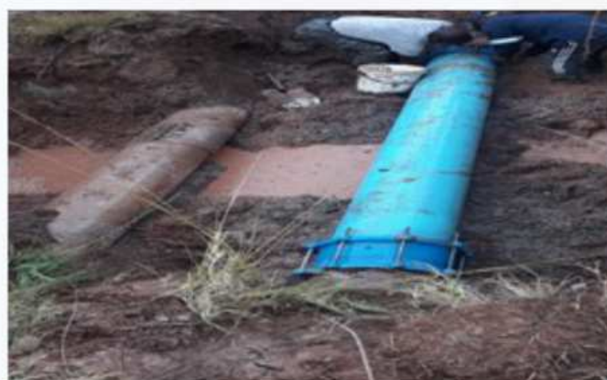
Repair of 350 mm pump line burst – Wilge Water Treatment Works
