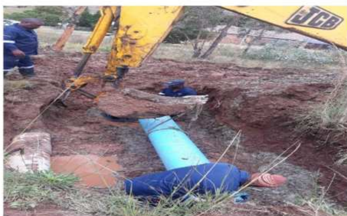
Repair of 350 mm pump line burst – Wilge Water Treatment Works
