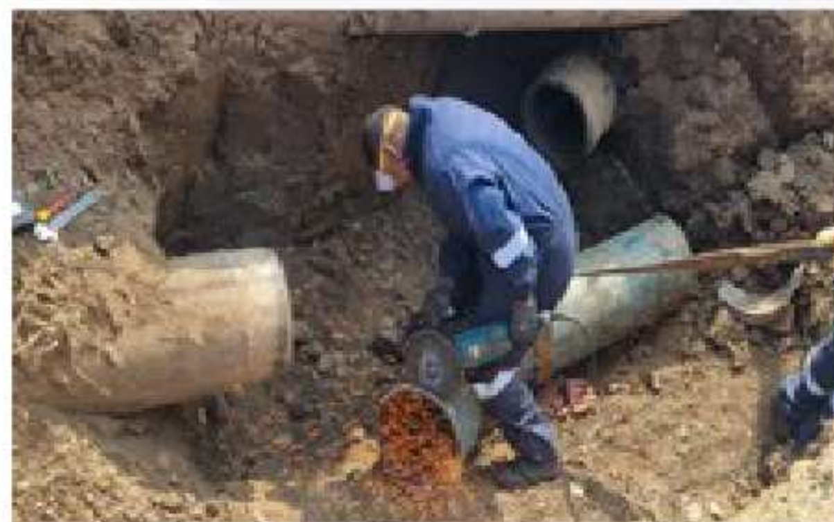
Repairs in progress
