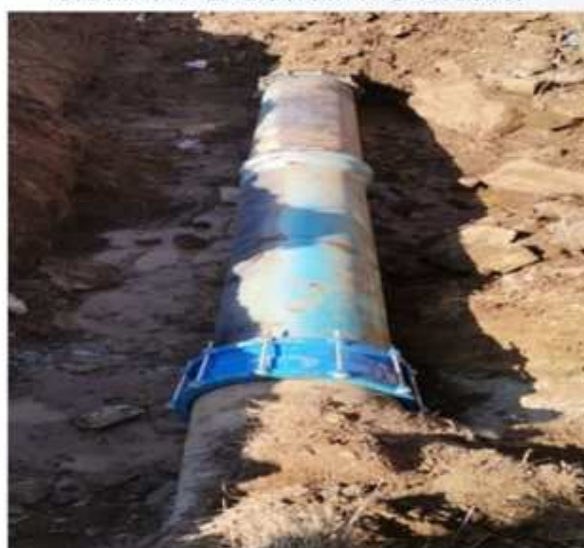
2 x 450 mm lengths of GRP pipe replaced with UPVC pipe
