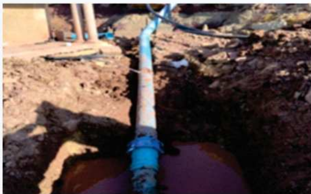
De Bult: Inlet pipe elbow burst – currently supported by temporary reinforcement. A new elbow, one UPVC pipe length, and a VJ coupling have been installed. A concrete slab is required for permanent support
