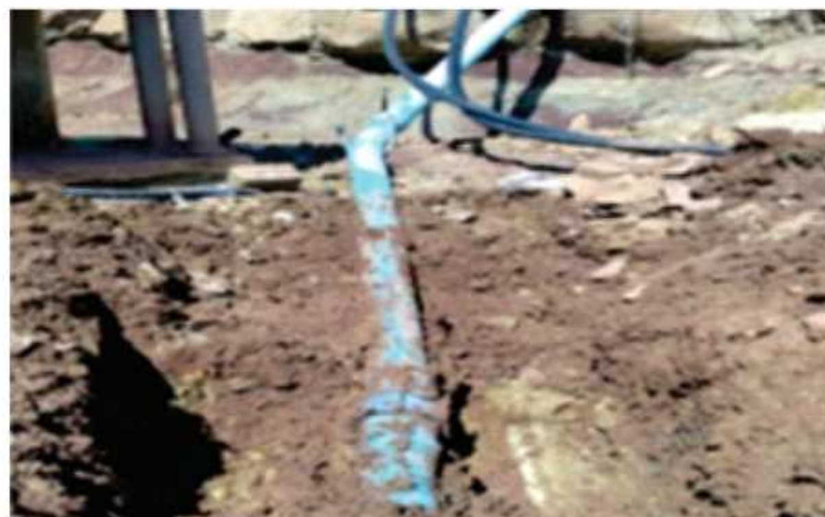
De Bult: Inlet pipe elbow burst – currently supported by temporary reinforcement. A new elbow, one UPVC pipe length, and a VJ coupling have been installed. A concrete slab is required for permanent support
