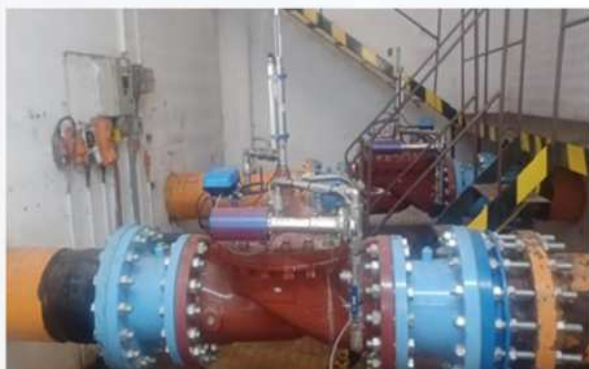
Installation of flow control valve at high lift pump station
