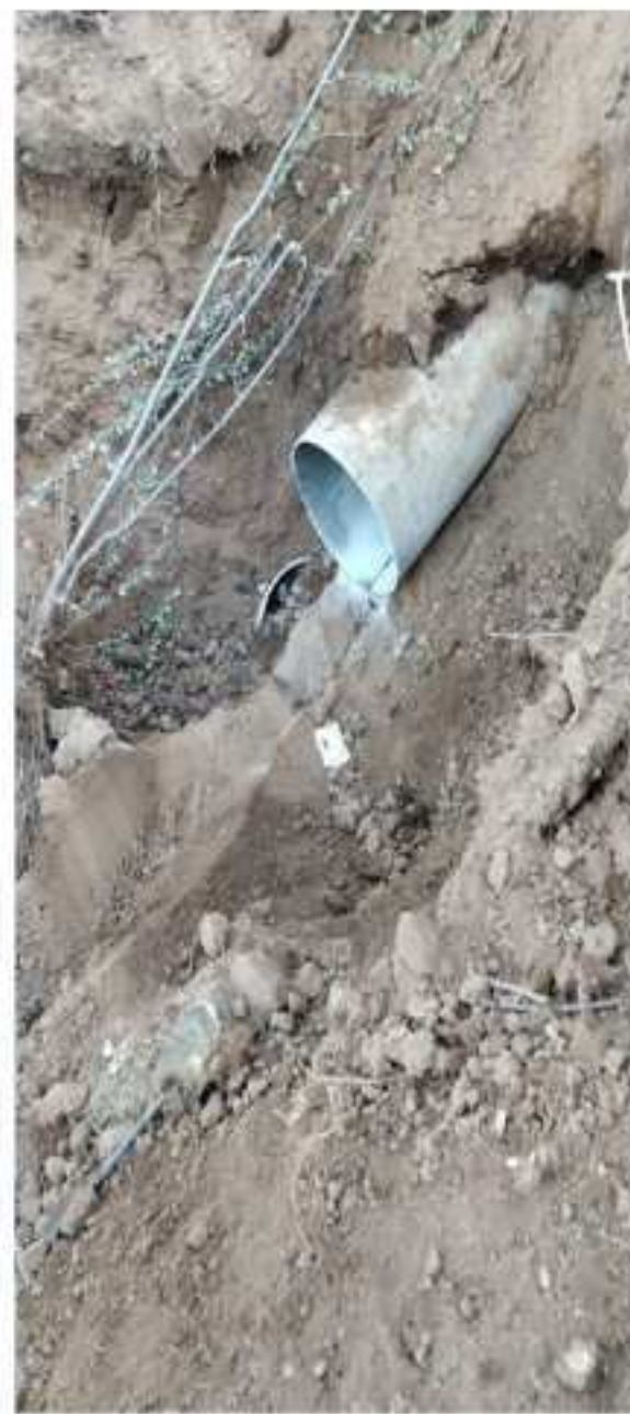
Repairing the GRP main supply line leakage
