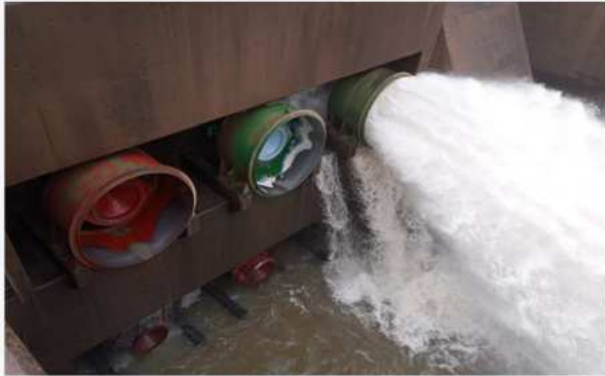
Welbedacht Dam – river outlet valves
