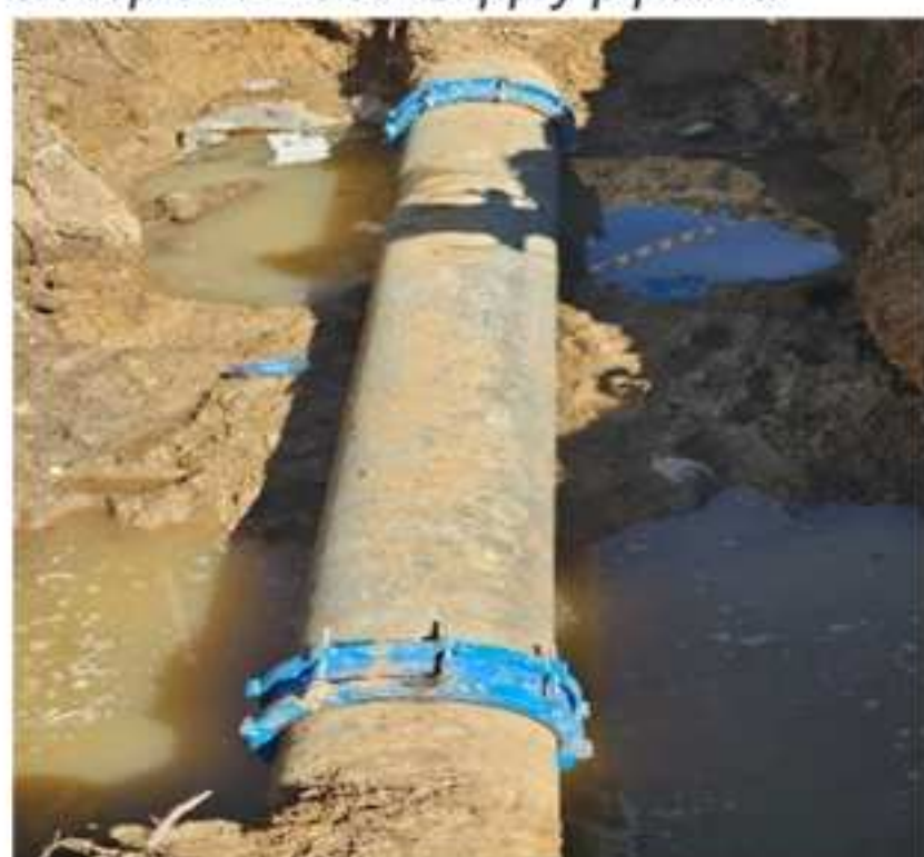
500 mm GRP burst replaced with a UPVC pipe
