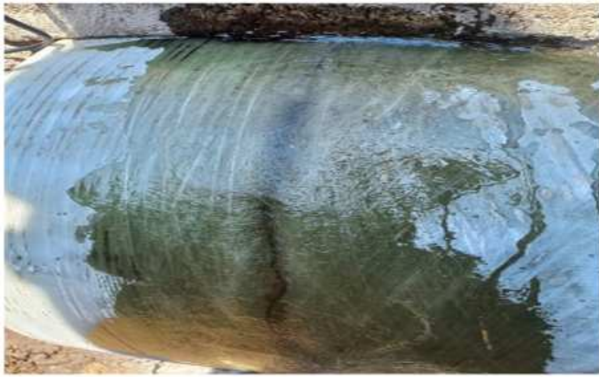
On-site adjustments made to scour the pipeline and repair the leaking GRP elbow after valves failed to close properly.
