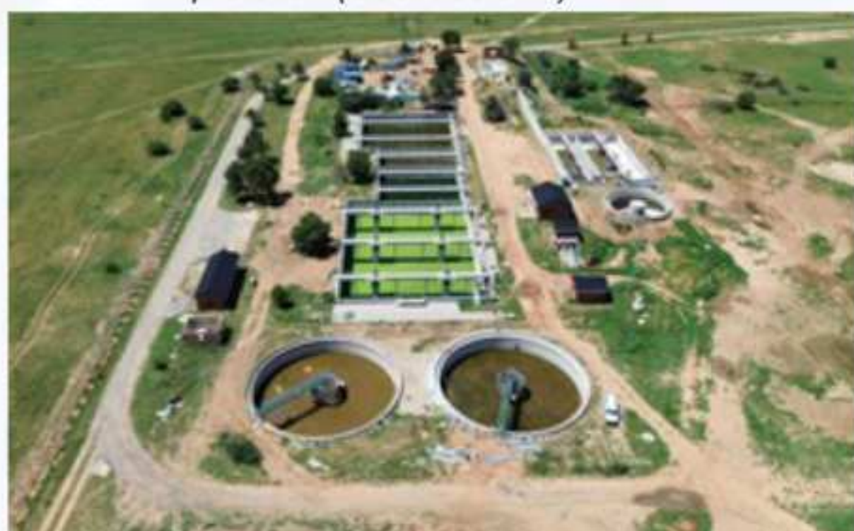
Kutlwanong Waste Water Treatment Works
