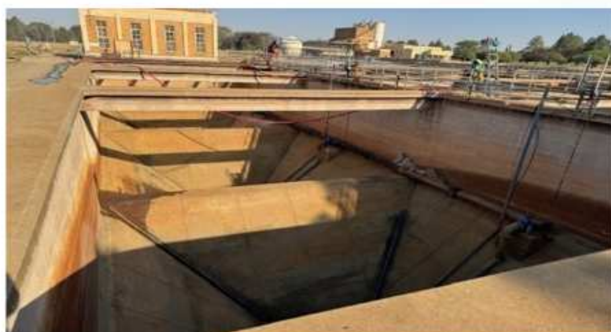
Cleaned settling dams
