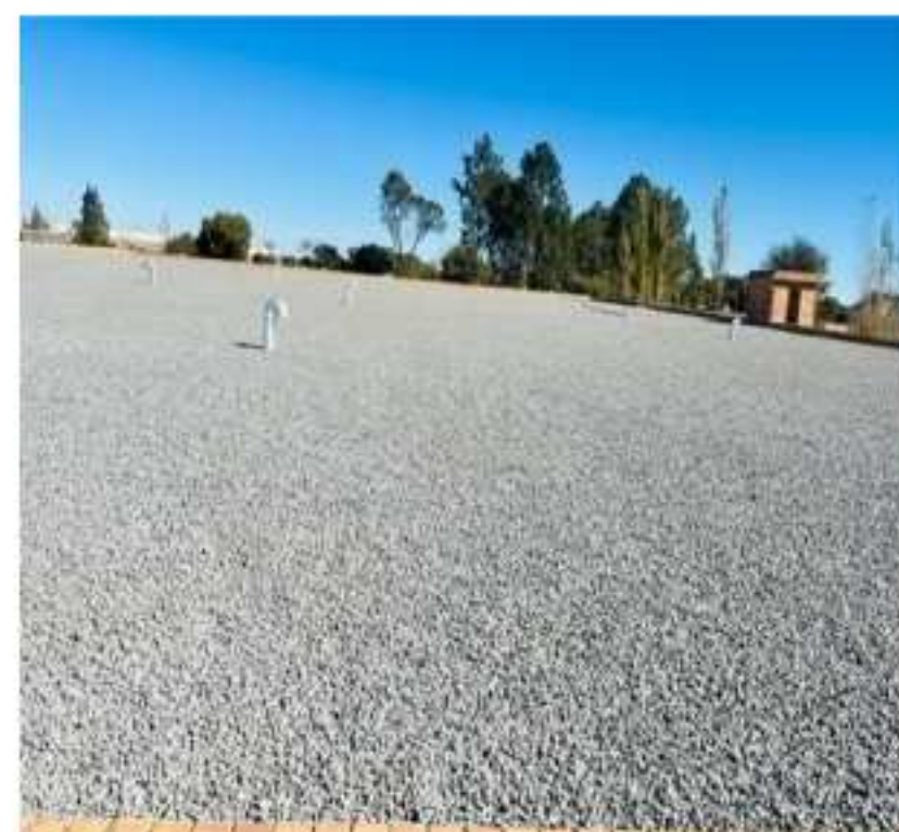
Allanridge Reservoir after refurbishment
