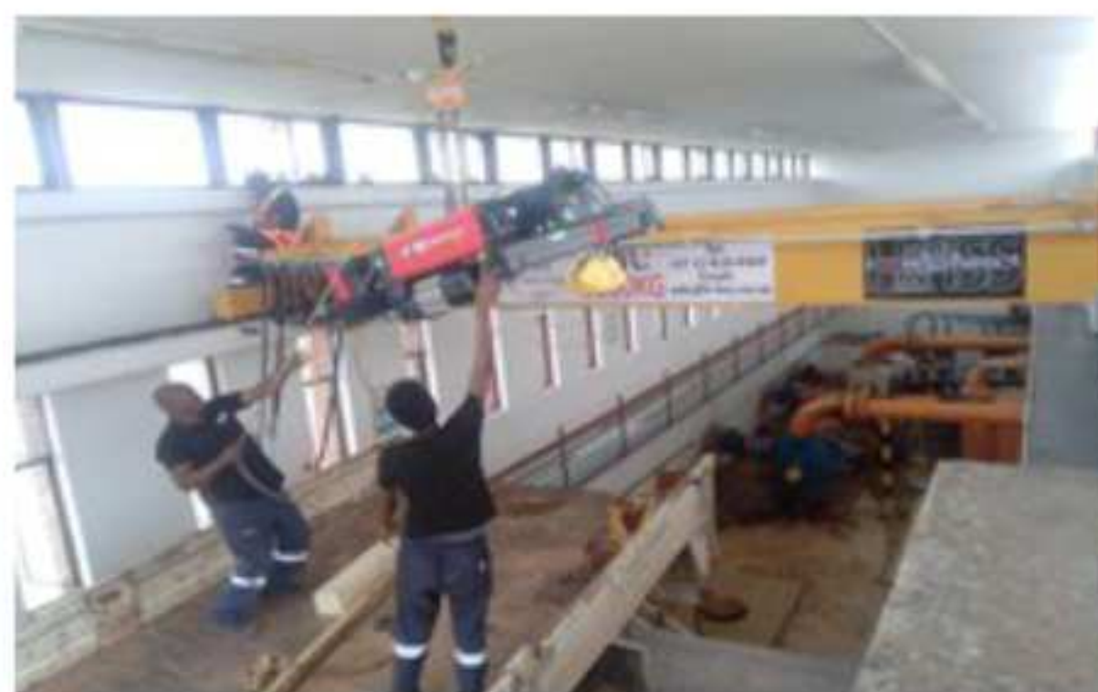
Installation of new overhead crane at Kneukel Pump Station
