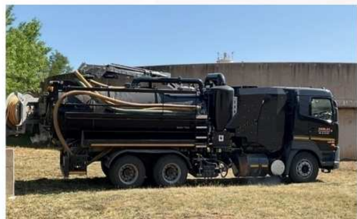
Drainpipe jet blasting between Turbo Circulator 2 and the filter plant
