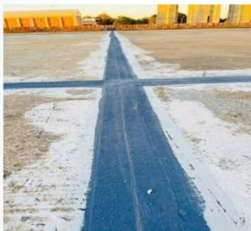
Expansion joints were repaired on the Allanridge Reservoir
