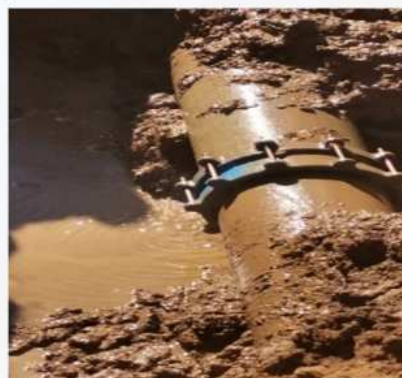
Repaired pipeline within a very dangerous, congested area
