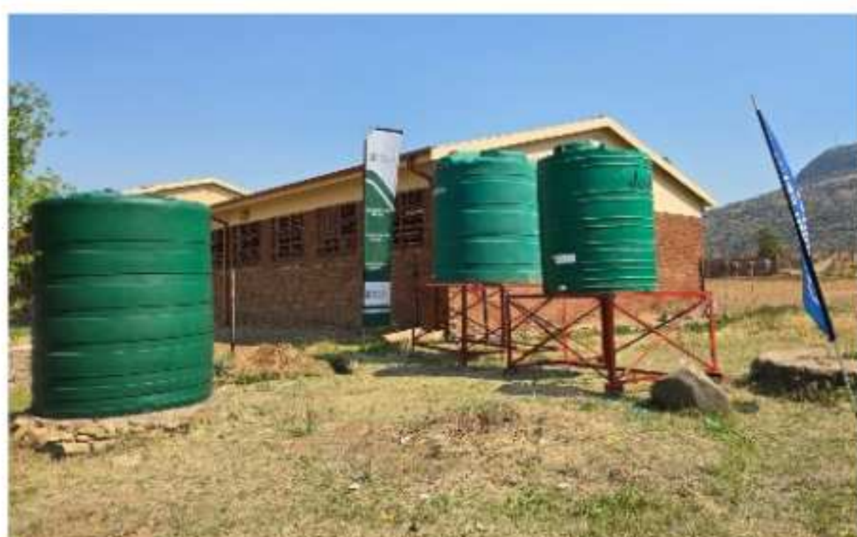
Vaal Central Water in partnership with Manguang Metro Municipality donated rain water harvesting tanks to Qibing Secondary School in Wepener
