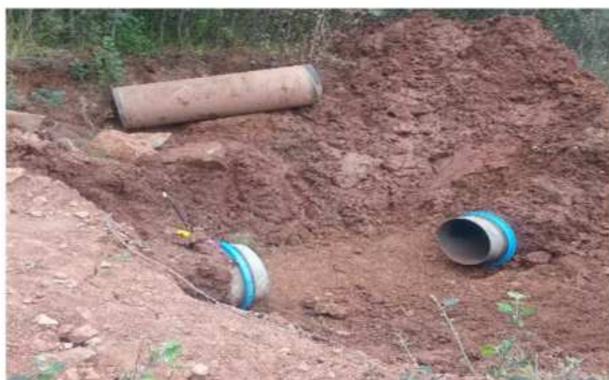
Fika Patso 700 mm GRP supply line burst
