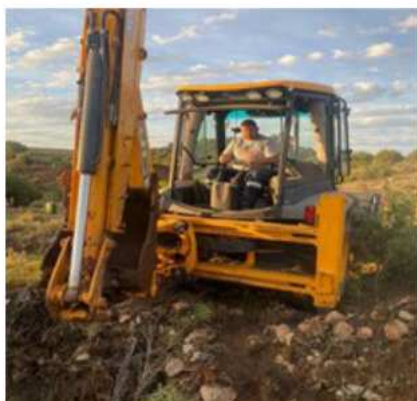
Maintenance on pipeline from Lemoenkloof to Jagersfontein Water Treatment Works
