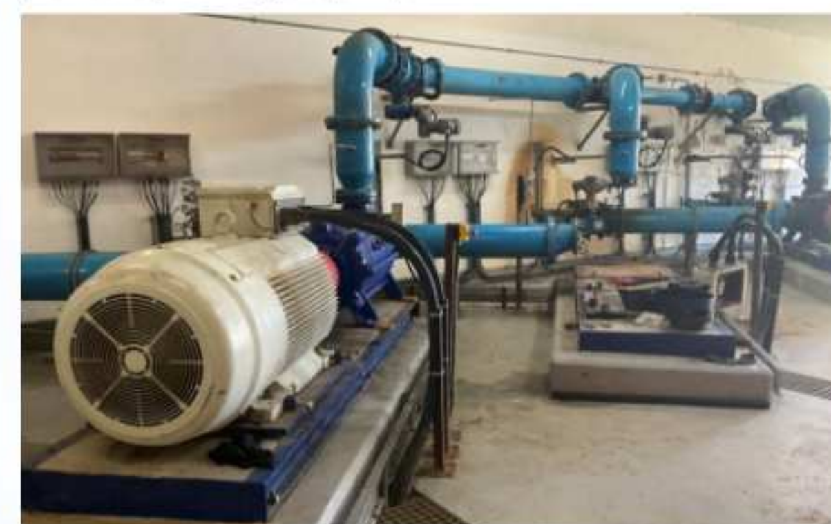
Intabazwe pump set removed for refurbishment
