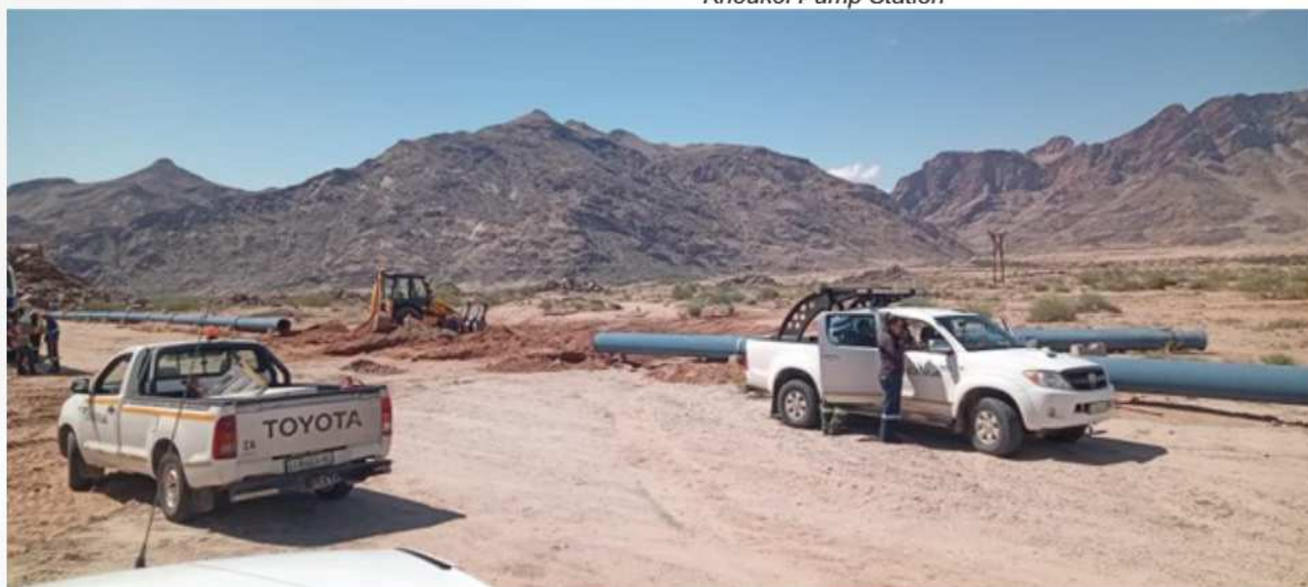
Repairs of the pipeline damaged by floods in Pella
