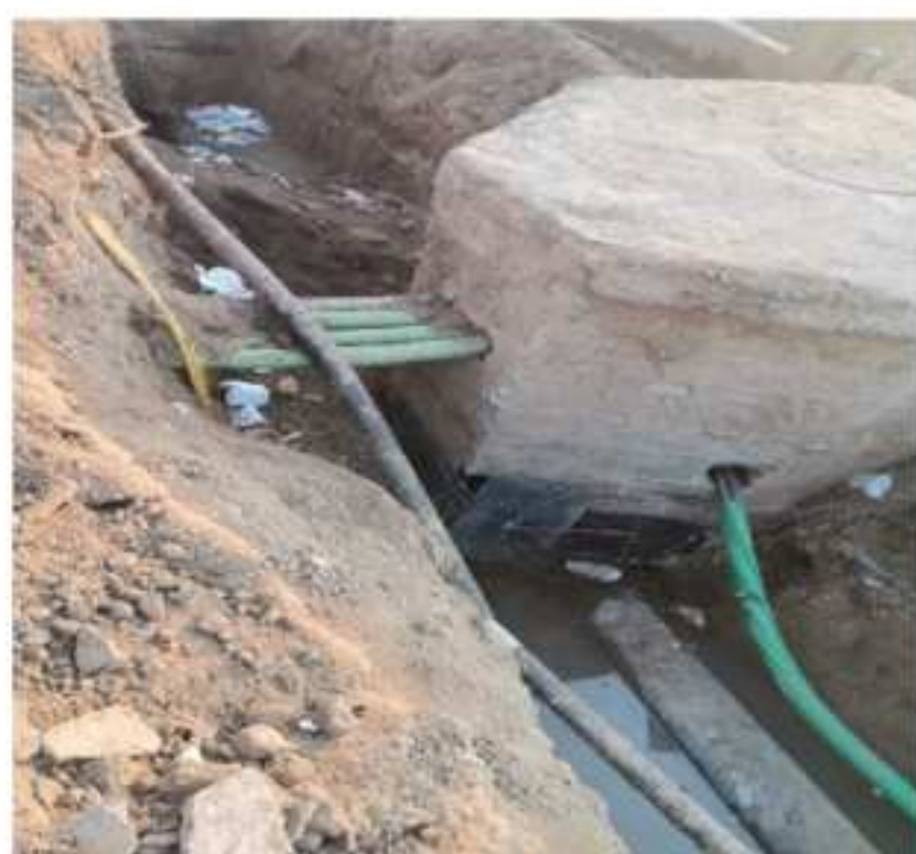
Telkom manhole chamber constructed on top of a water supply pipeline
