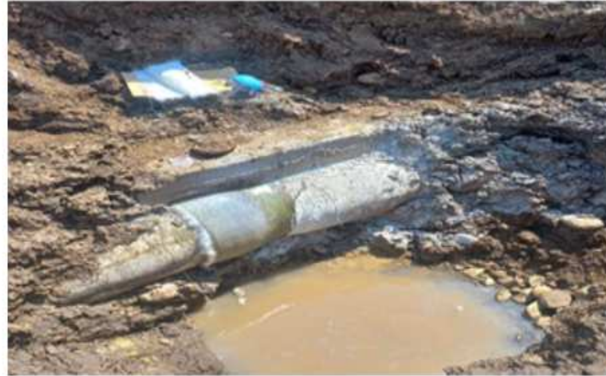
Repairing the damaged 700 mm GRP pipe at Thabatshweu
